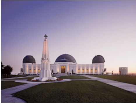
Photo © Tim Griffith
